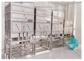
Figure 5. Palletank skid for buffer storage with stainless steel piping headers for filling and distribution, located in buffer preparation room.
