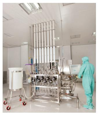
Figure 7. Buffer distribution skid in process room, with flexible hoses directly connected to chromo system and to drum bag for filling.
